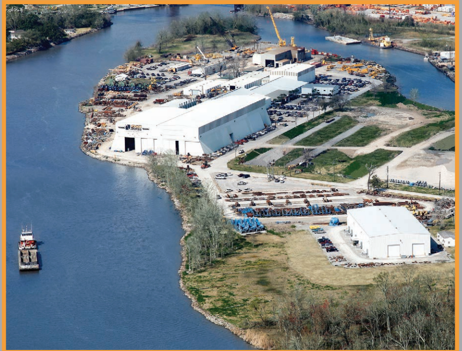
Oil States Skagit SMATCO's 185,000 square foot manufacturing, engineering, sales and service facility with waterfront access.
