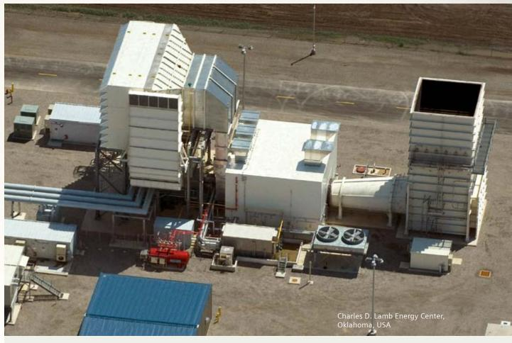
SGT6-2000E Heavy-duty gas turbine
